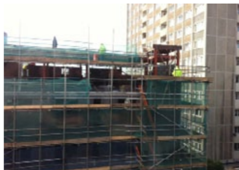
伦敦 Central Street 酒吧改建成 8 套公寓——施工中 8 apartments to replace a pub in Central Street, London EC1-Under Construction
